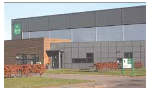
DLH, new plywood factory, Kolding.
